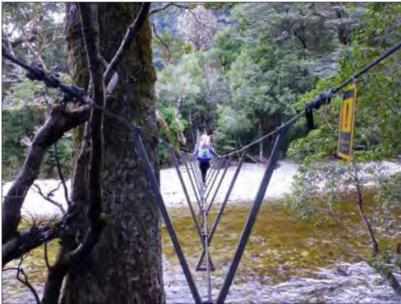
Cathye on a three-wire bridge over the Wapiti River
