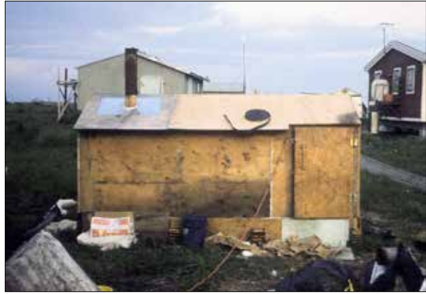
A backyard meqiq or wash-house for the family since there was no running water in the village
