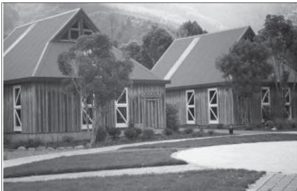
Anakiwa Outward Bound Bunkhouses
